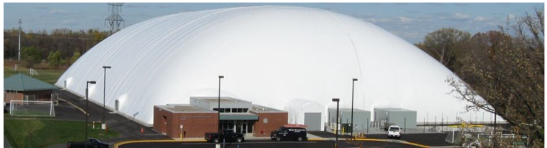
Maple Grove Sports Dome (200'x400') City & High School partnership
